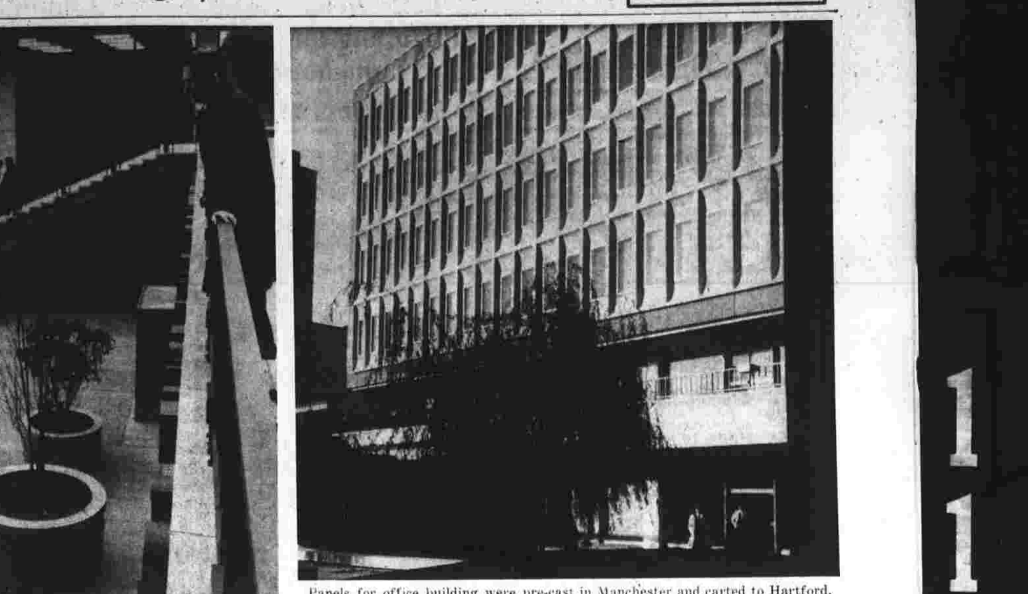
Panels for office building were pre-cast in Manchester and carted to Hartford.
